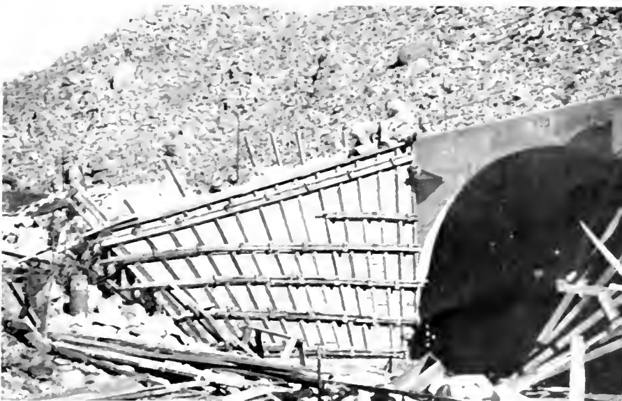
FIG. 34. Construction of warped end wall
